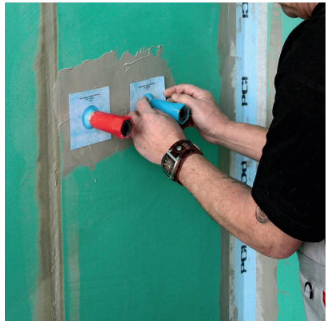
2. PCI Pecitape 10 x 10 is placed over the pipe connection protruding from the wall and covered with PCI Lastogum (gray).
