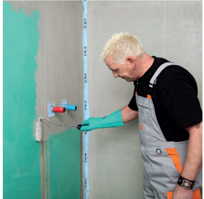
4. Apply undiluted PCI Lastogum (gray) to the substrate as a first protective layer covering the entire surface.
