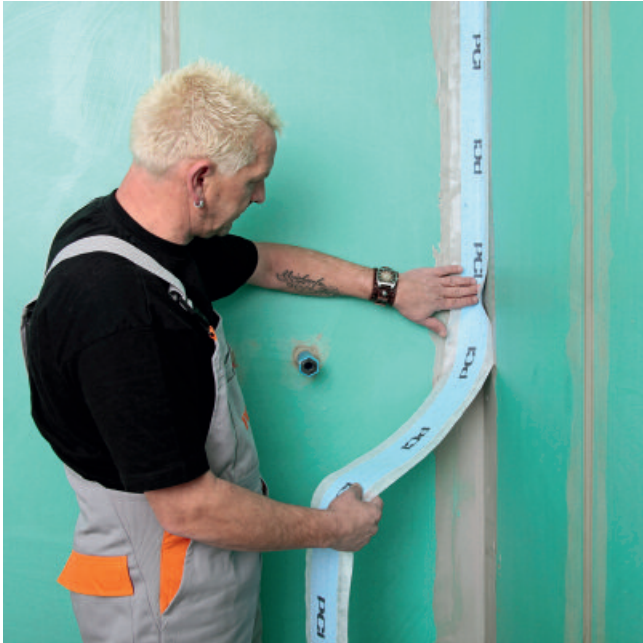
3. PCI Pecitape120 fixed with PCI Lastogum (gray) in corner joints and floor/wall junctions.
