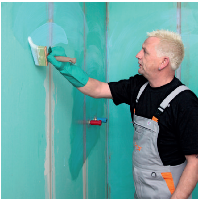
1. Absorbent mineral substrates or gypsum-based substrates and plasterboards primed with PCI Gisogrund.
