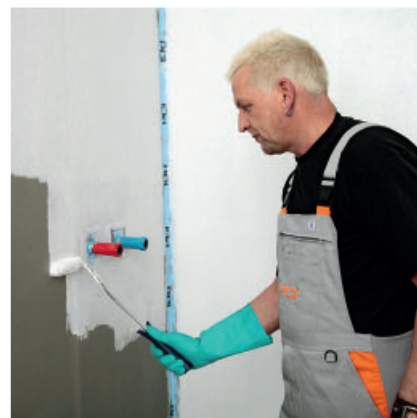
Undiluted PCI Lastogum applied to the substrate by roller, brush or trowel.
