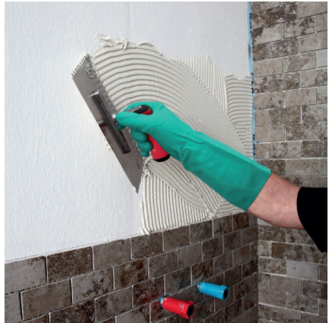
6. Allow the waterproofing layer PCI Lastogum to cure before laying tiles and flagstones.
