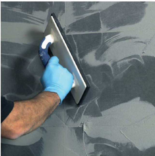
Workable grouting within approx. 40 minutes.
